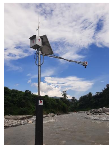
Photo of a Ground Sensor Terminal installed in Melamchi River for Flood Early Warning System ©APN
