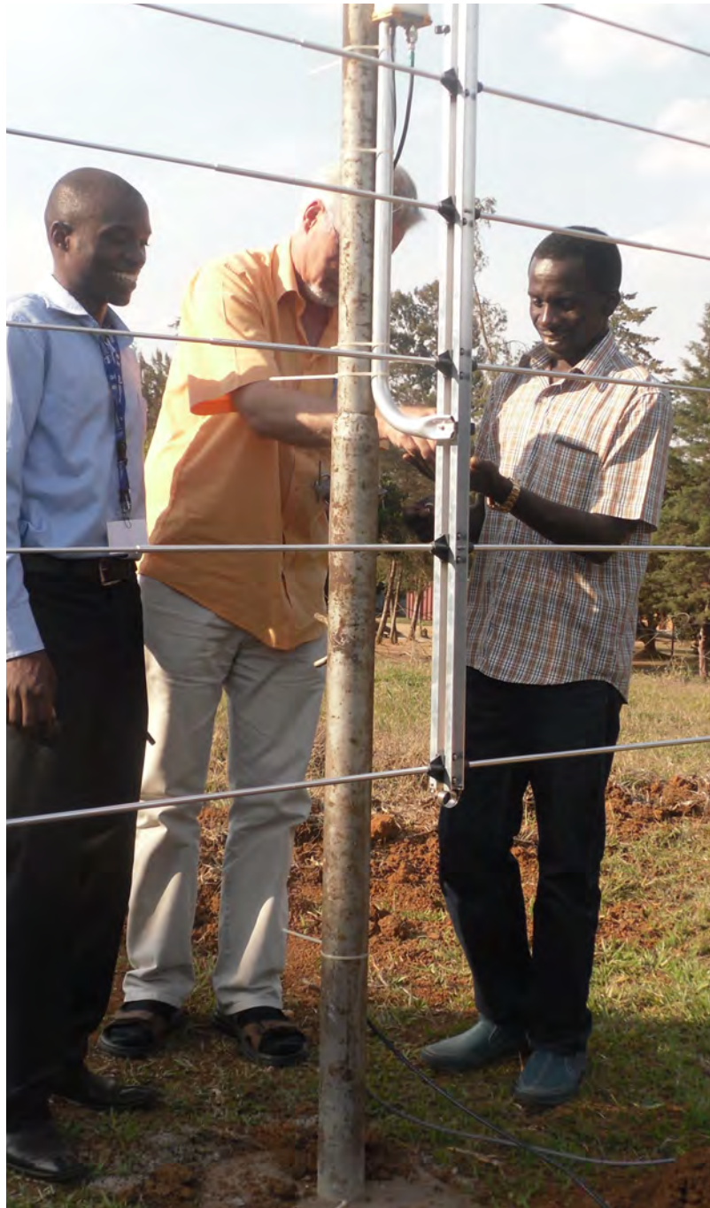
Advancing Space science research and education through instruments deployment: Here installation of a CALLISTO solar spectrometer at the University of Rwanda
